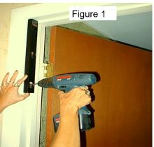
should be taken into consideration when deciding which set of holes in the bracket to use. Expand the bar until it is tight between the door frames. The bar must be tight between the brackets but it may be possible to crack the door frame by over tightening.
