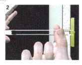
Hold ends of straps between thumb and forefinger and pull toward you until channel rests flush behind wall. Slide plastic cap along straps with other hand until flange of cap is flush with wall
