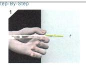
Drill a 1/2" (Ø13mm) hole. Hold metal channel flat alongside plastic straps and slide channel through hole. Minimum clearance behind wall: 1-7/8" (48mm).
