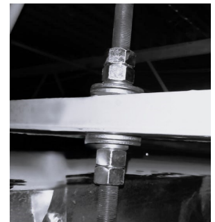
Figure 8 Threaded Rod Bottom End Hardware Attachment Order Detail:
